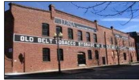
Luna nanoWorks renovates a tobacco warehouse for nanomaterials manufacturing and R & D.
